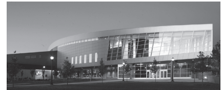
Spokane Convention Center Group Health Exhibit Hall which just earned Silver LEED Certification from the U.S. Green Buildings Council. Photo credit: Spokane Convention Center
